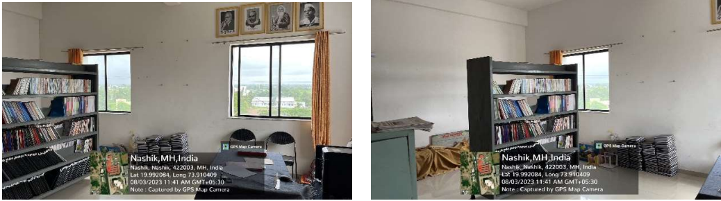
Effective use of day lighting by orientation of building; ample day light in the reading areas
